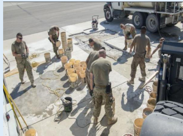
Bagram Airfield, Afghanistan: 405th Expeditionary Support Squadron Civil Engineers execute rapid spall repairs exercise.
